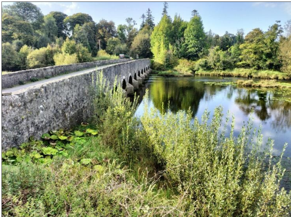
Plate 14.10: View of Palmerstown Bridge
